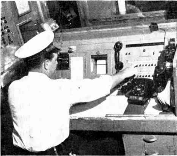
Alarm system looks for trouble
