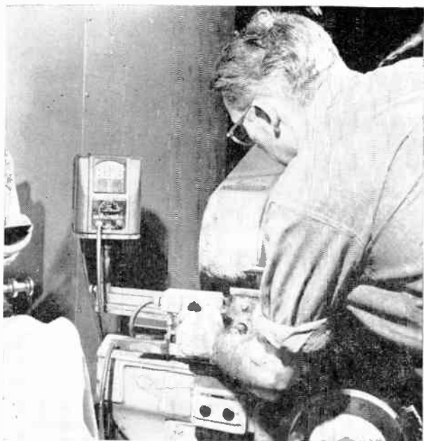
Amplifier picks up piston taper
