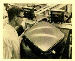
Zenith engineers new 25-inch three-gun color picture tube with 90-degree deflection.
