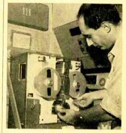
Motion pictures are transmitted from the Sony video tape machine located in cockpit of American's 707 and 720 Astrojets. Astrovision, a four-part in-flight entertainment system, also features stereophonic classical and popular music, live and tape TV, and in-flight photos.
