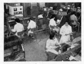
TRANSISTOR PRODUCTION is carried out in "dry boxes" to exclude dust and moisture. Operators work through gloves. Insides must be clean.
