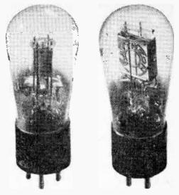
FAMOUS FIRST is this Type 27, believed to be the earliest of the indirectly heated cathode types (left) and Type 71, a directly-heated cathode type circa 1926. Note the addition of the base.
