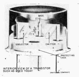
INSIDE A RAYTHEON transistor, we see the contact terminals and the supparts far the fusian-allay base.
