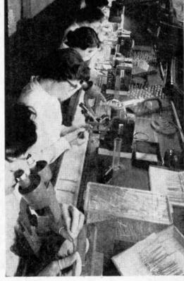
ASSEMBLING SUBMINIATURE tubes is done under microscopes. Each operator is equipped with microscope and miniature welder. Note rubber fingers.
