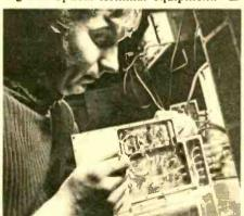
One of the two repeaters that is used along six mile route to boost and reshape the infrared pulses that are transmitted along the optical fiber. An engineer is seen here making final adjustments to this repeater before installation in the optical link between Stevenage and Hitchin.
