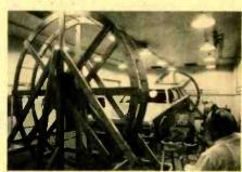
A new 1978 stationwagon is tested for effects by outside power line radiation. GM also measures RF noise generated by auto.
