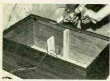
Glue around edge of cabinet, don't leave any gaps. Wire up the midrange enclosure.
