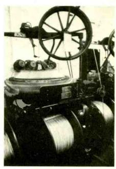
A patent weaving machine is used to spin the shielding braid around the foam dielectric in this photo from Alpha Wire Corp.
