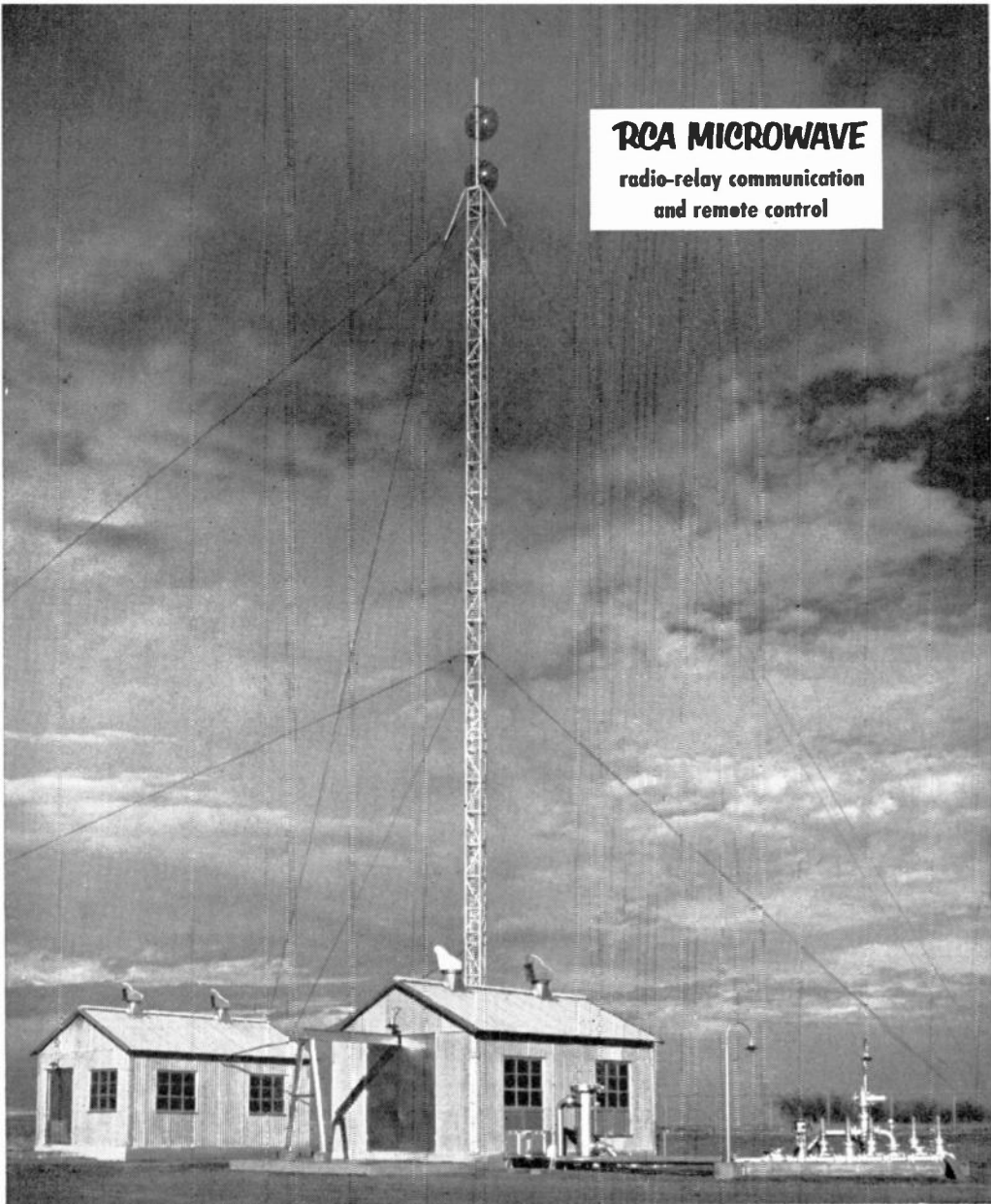
Unattended booster station at Pernell, Okla. Radio-beam signals via RCA Microwave operate the booster
