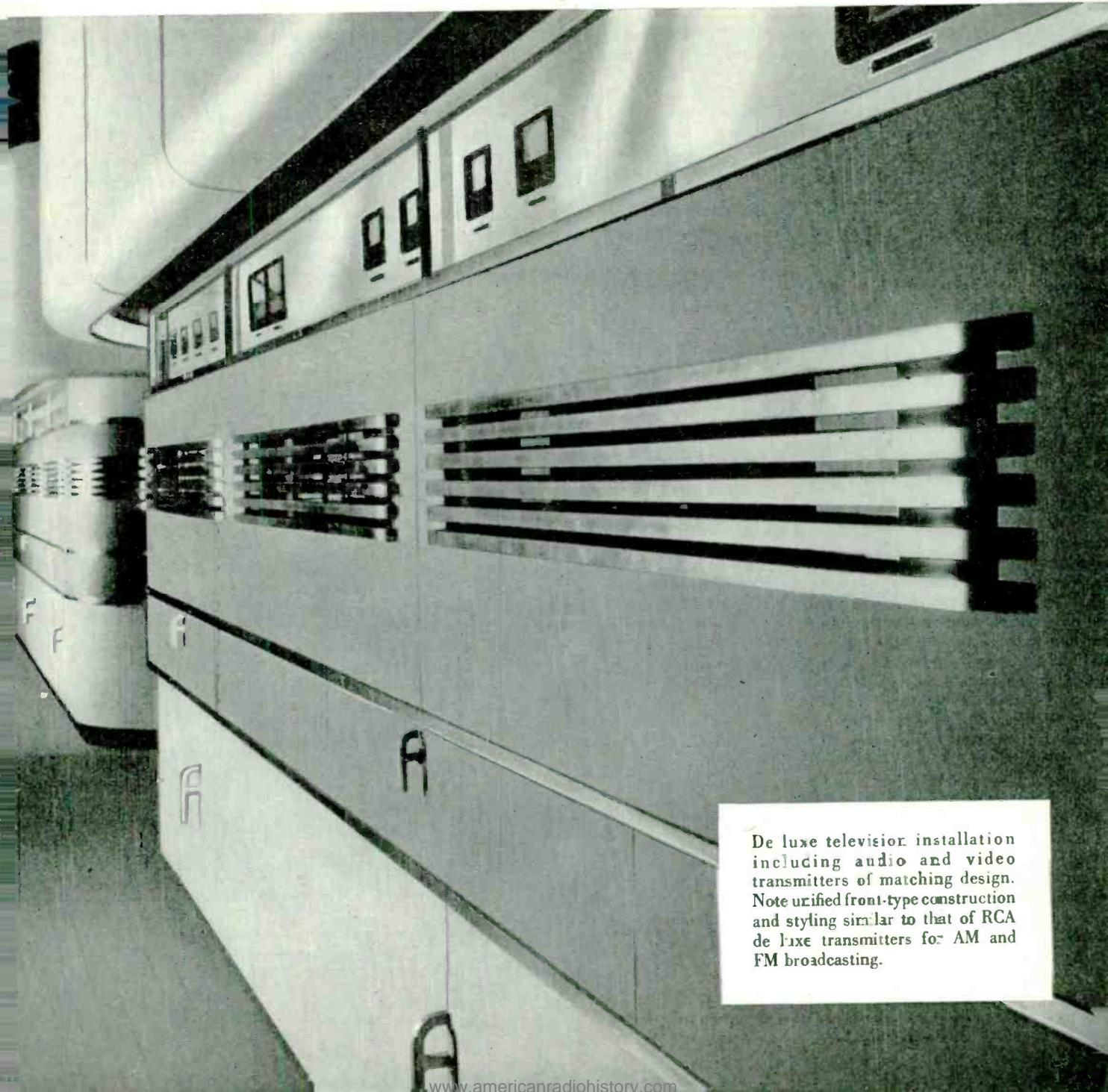
De luxe television installation including audio and video transmitters of matching design. Note unified front-type construction and styling similar to that of RCA de luxe transmitters for AM and FM broadcasting.
