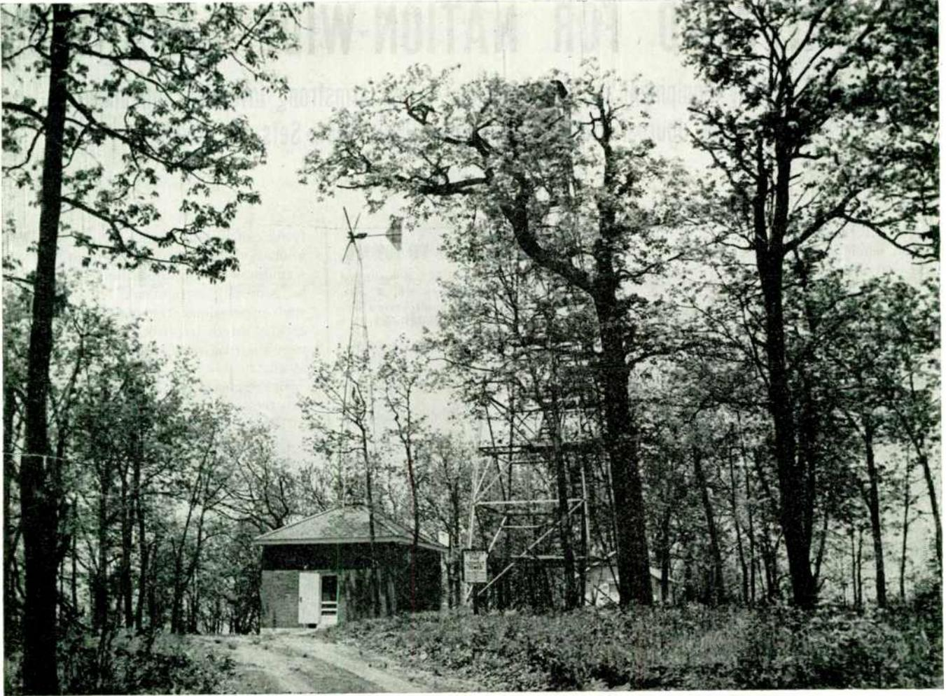
FIG. 1. WINCHARGER AND EMERGENCY ENGINE-DRIVEN GENERATOR POWER THIS REMOTE FM RELAY INSTALLATION
