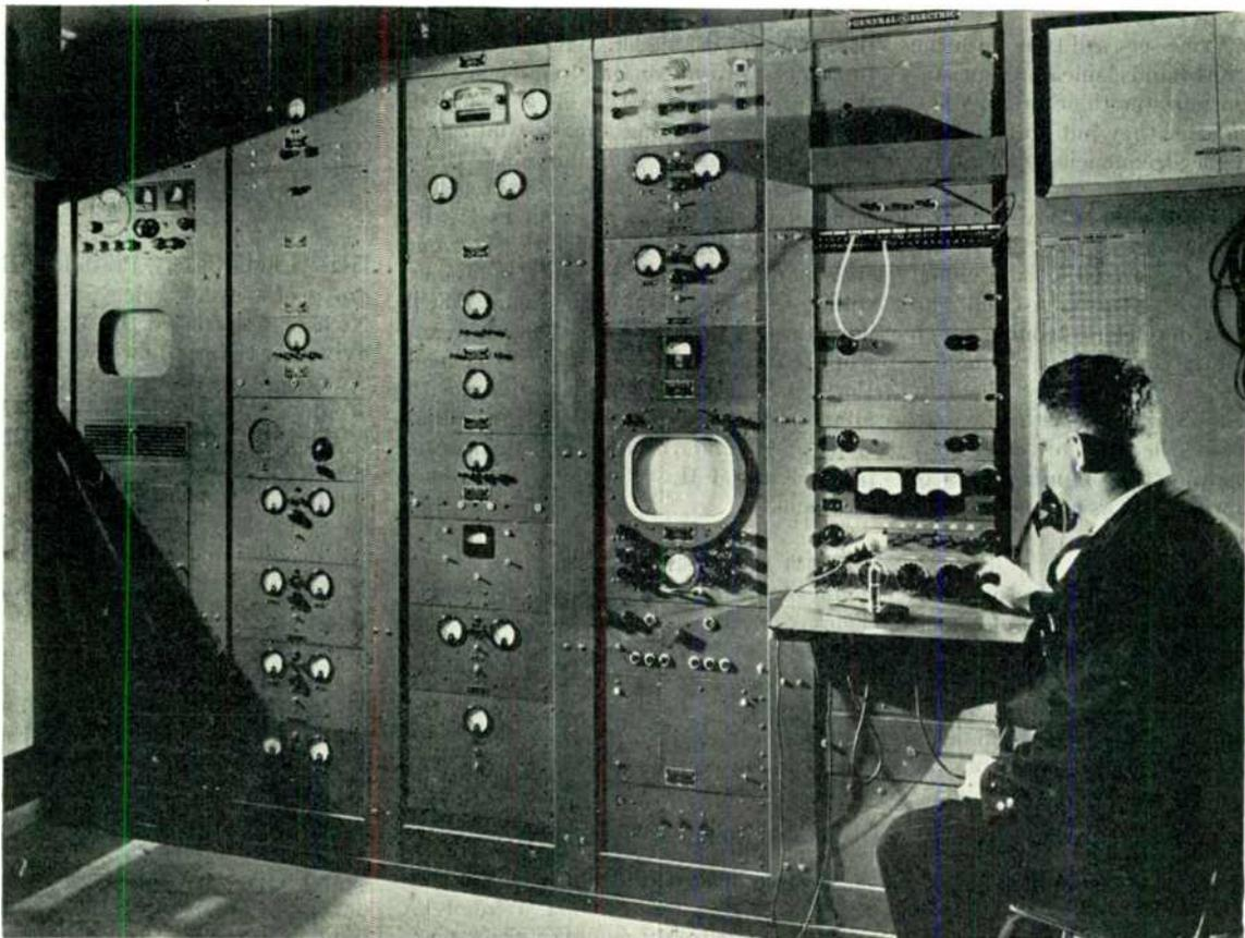
FIG. 40. RECEIVING, MONITORING, AND TRANSMITTING EQUIPMENT THROUGH WHICH WNBT SIGNALS GO TO WRGB
