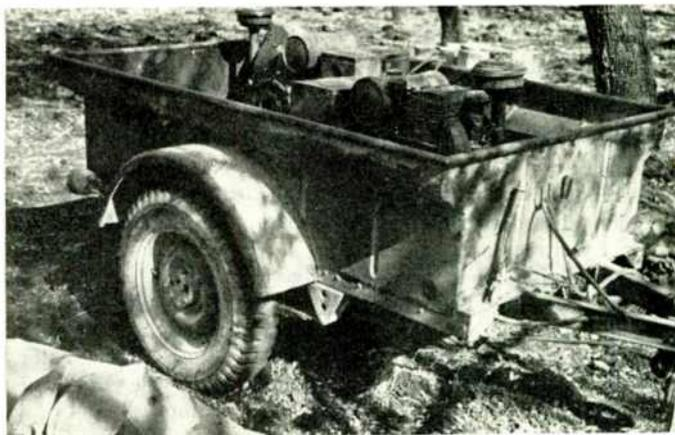
POWER SUPPLY FOR A MOBILE FM STATION WAS CARRIED IN A LIGHT TRAILER, AND HAULED BEHIND RADIO TRUCK
