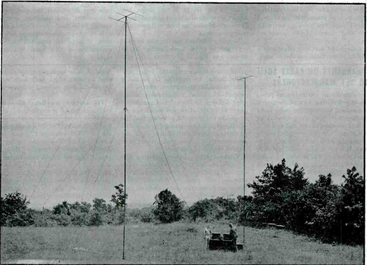
FIG. 10. 3-ELEMENT HORIZONTALLY POLARIZED ANTENNAS USED FOR MILITARY RELAY PURPOSES ON 70 TO 100 MC
