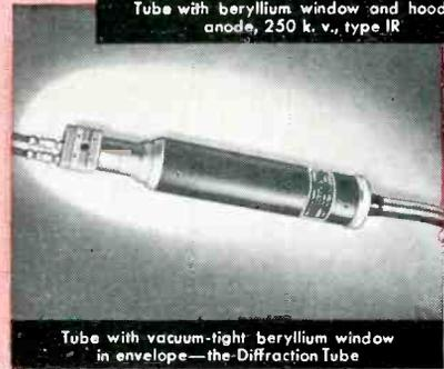
Tube with vacuum-tight beryllium window in envelope—the Diffraction Tube
