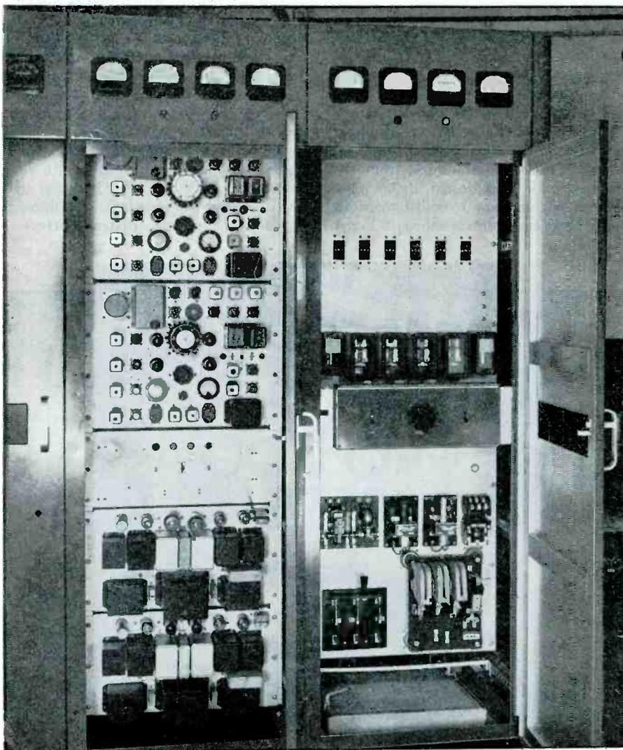
FIG. 7. CENTER UNIT OF THE 8-KW. TRANSMITTER CONTAINS A SPARE EXCITER
