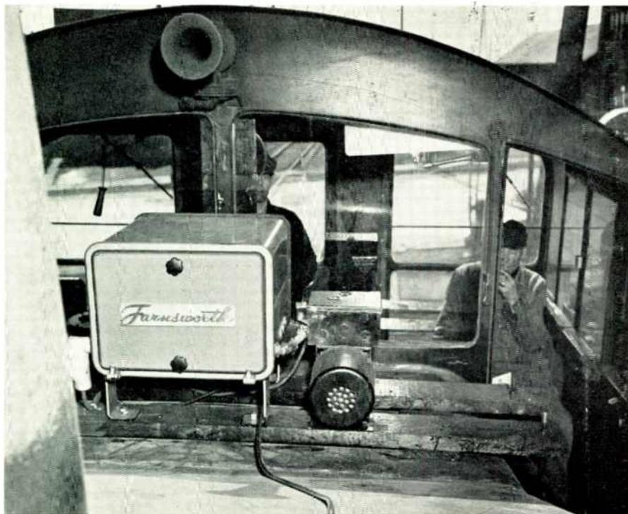
FIG. 11. THIS SHOWS THE METHOD OF MOUNTING THE RADIO EQUIPMENT ON A DIESEL ENGINE. THIS VIEW IS LOOKING INTO THE CAB FROM THE FRONT
