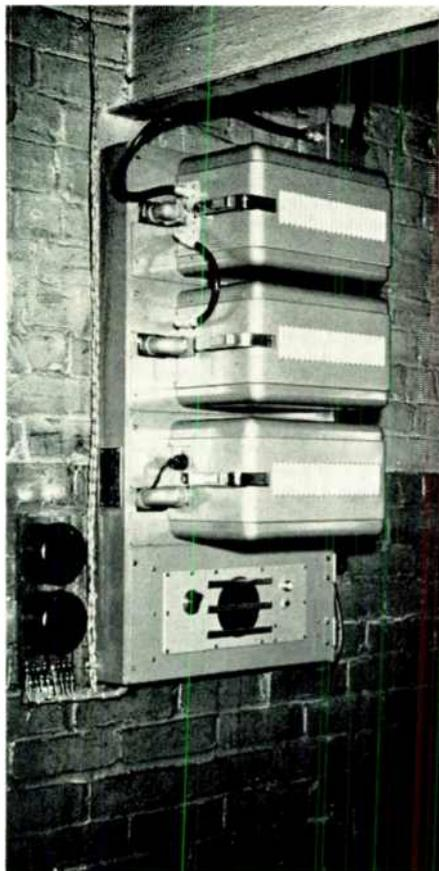
FIG. 8. INDUCTION RECEIVER AND TRANSMITTER AT MICHIGAN CENTRAL TOWER
