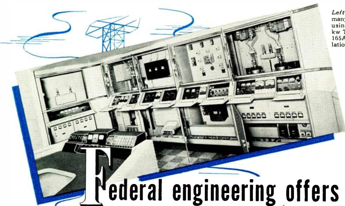
Left: WDOD is one of many network stations using Federal's five kw Transmitter, Type 165A, a pre-war installation.
