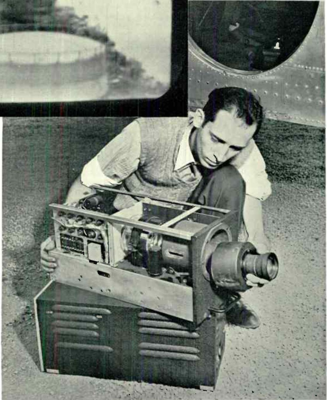
AIRBORNE TELEVISION EQUIPMENT USED FOR OBSERVING ENEMY TERRITORY FROM THE GROUND. IT IS CARRIED IN SCOUTING PLANES OR RADIO-CONTROLLED SHIPS
