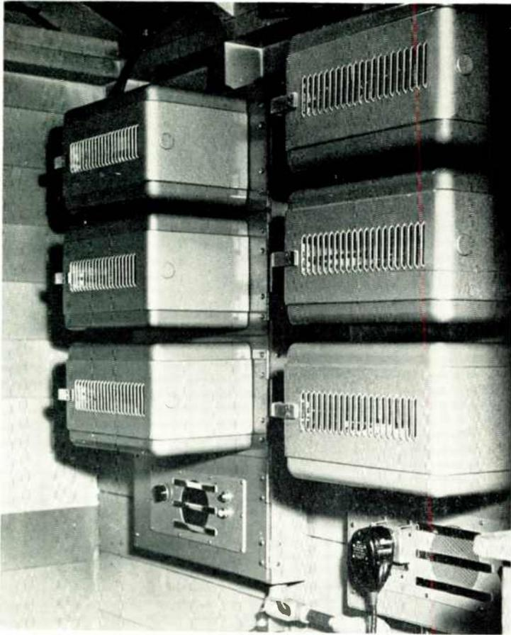
FIG. 4. POWER SUPPLY, TRANSMITTERS, AND RECEIVERS FOR FM INDUCTION AND SPACE RADIO AT THE FLAT ROCK MAIN STATION
