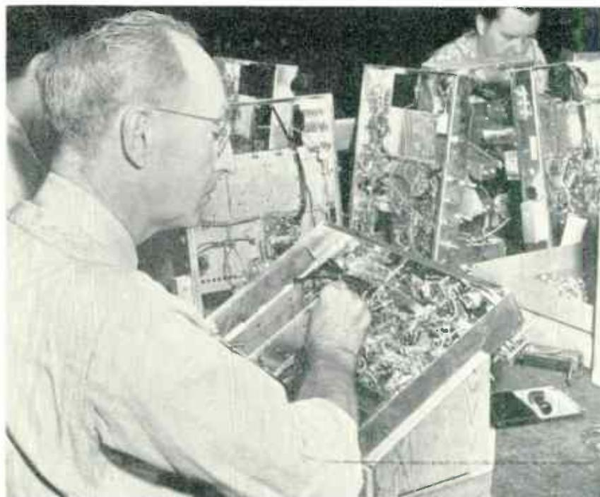
7: WORK IS DISTRIBUTED IN UNITS OF TIME, TO KEEP LINE MOVING STEADILY. 8: FREQUENT INSPECTION CATCHES ERRORS QUICKLY
