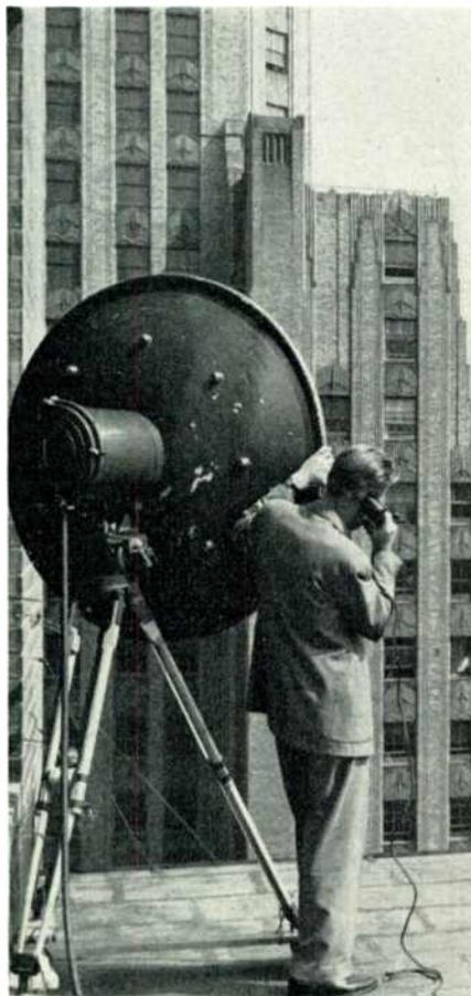
FIG. 1. MICROWAVE TRANSMITTER FOR TRANSMITTING A TELEVISION PROGRAM FROM THE WALDORF TO WNBT
