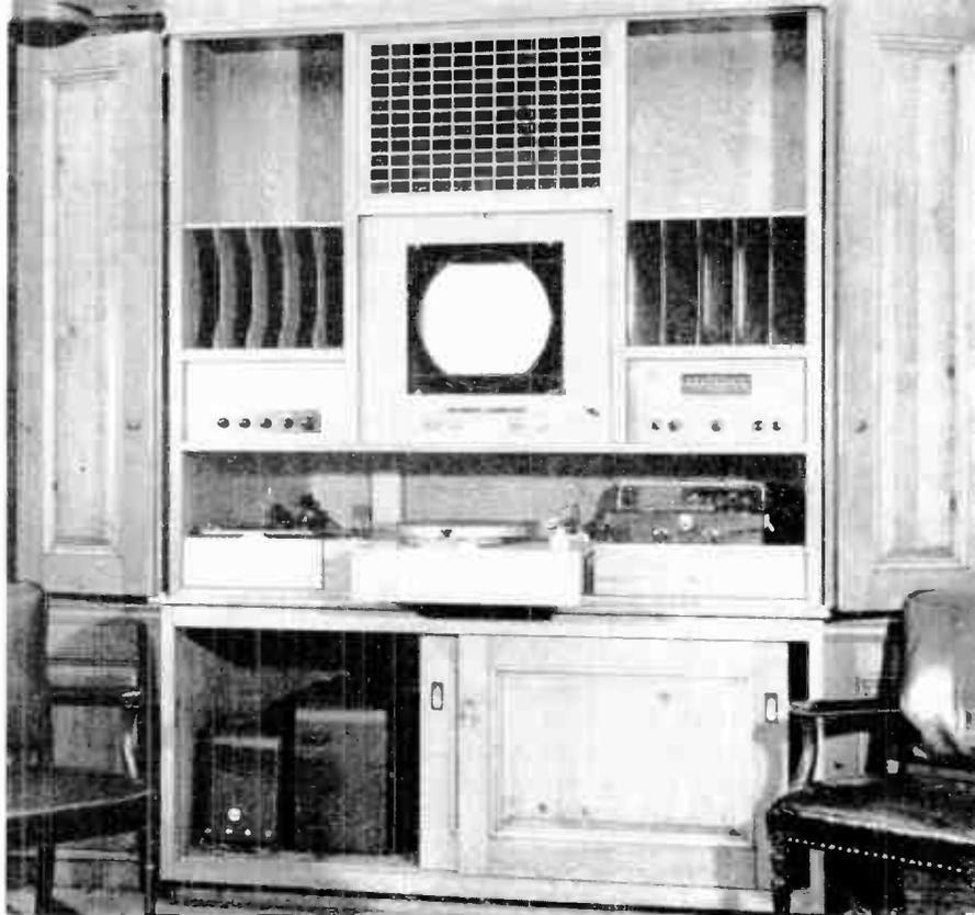
*Figs. 7 and 8. Another cupboard installation. Individual units can be replaced easily as they become worn or obsolete*
