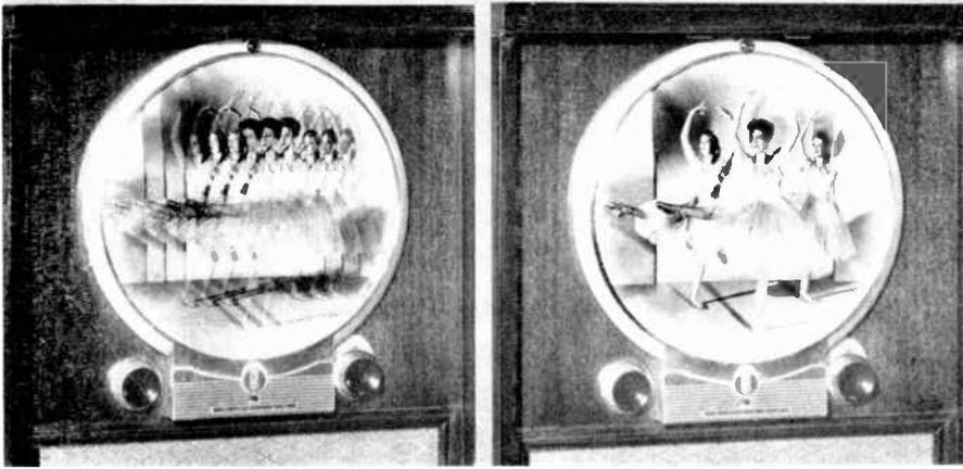
*Figs. 1 and 2. Phonevision reception before and after addition of the key signal*
