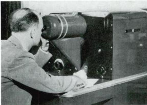
DR. C. H. BACHMAN AT THE EYE-PIECE OF NEW ELECTRON MICROSCOPE DEVELOPED BY GENERAL ELECTRIC. ENLARGEMENT IS 10,000 TIMES. VOLTAGE VARIATIONS DO NOT AFFECT MAGNIFICATION
