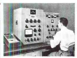
This test position involves two practical problems in a precision inductor. The unit shown is adjusted to an inductance accuracy of .3%, with precise (high) Q limits. It is then oriented in its case, using a test setup which simulates the actual final equipment so that minimum inductive coupling will result when installed in the final equipment,
