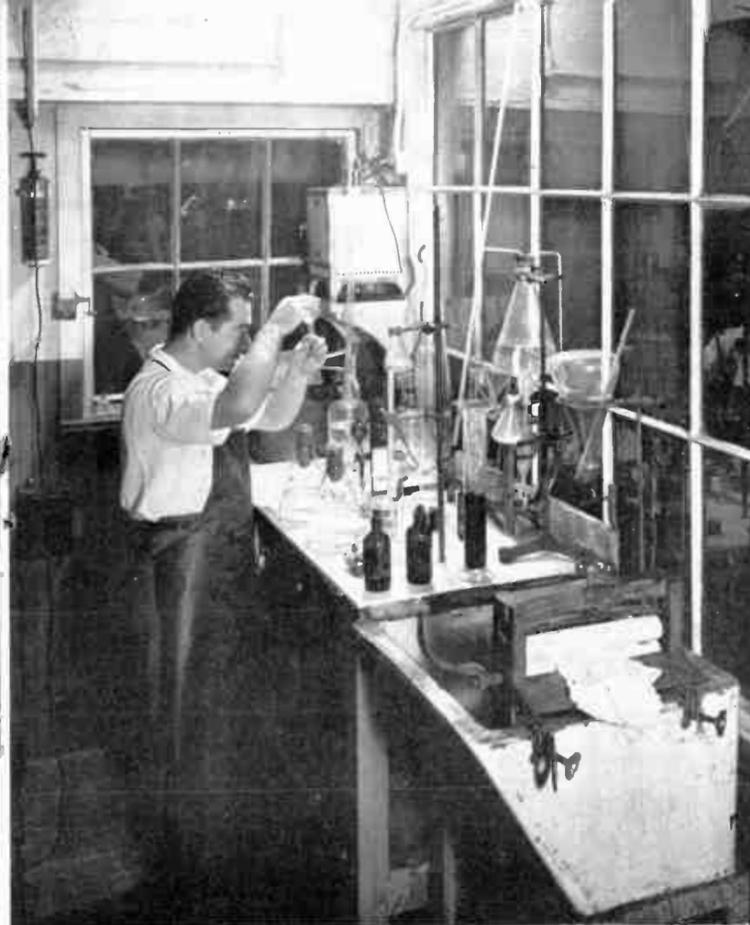
FIG. 5. RESIDUAL BLEACH WOULD CONTAMINATE THE FINISHED PAPER. THE BLEACH CONTROL CHEMIST CHECKS THE STOCK
