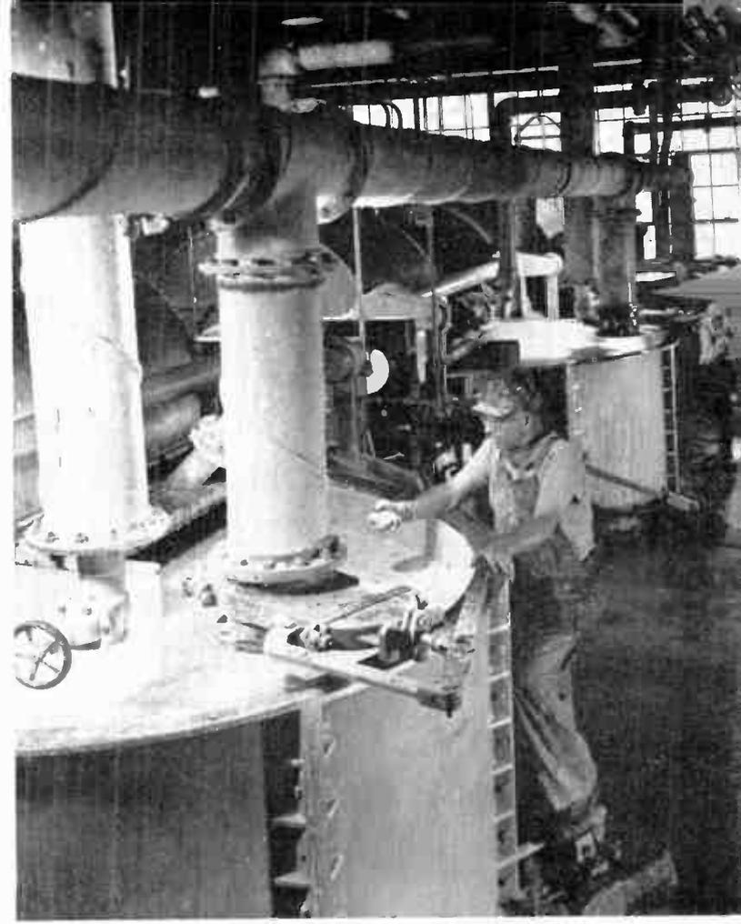
FIG. 6. THE FIBRE IS FURTHER SHORTENED IN THE BEATER, FROM WHICH IT GOES TO THE PAPER MACHINE
