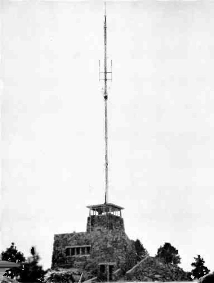
FIG. 4. THE 125-FT. ANTENNA ON MT. COOLIDGE. BEAM ARRAYS ARE FOR COMMUNICATION WITH RAPID CITY
