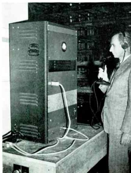
BELOW: FIG. 4, LEFT, ONE OF THE INTERMEDIATE AMPLIFIER POINTS BETWEEN THE STADIUM AND THE RACE STREET TERMINAL
