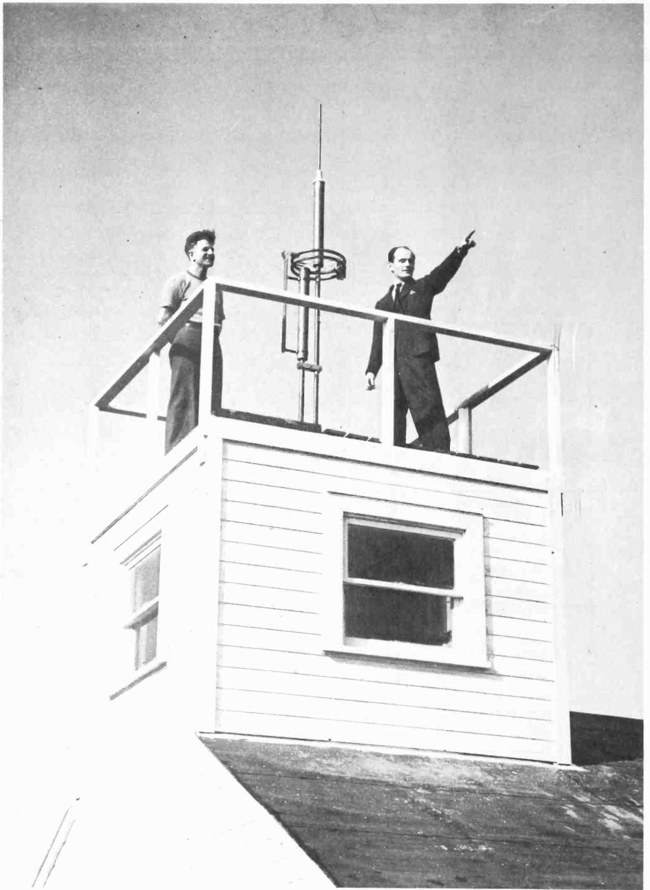
Fig. 3.—Circular polarization antenna.
