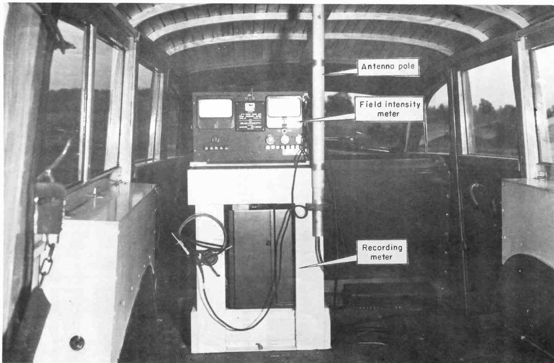
Fig. 11. — Field intensity measuring installation in field car.
