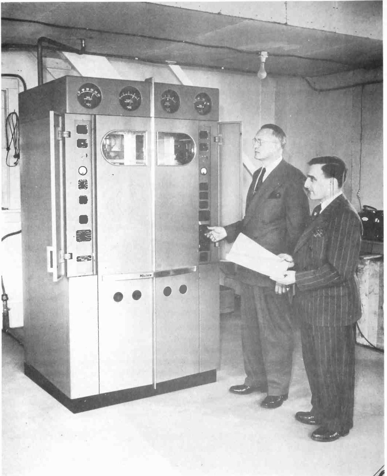
Fig. 2.—Western Electric 1kw type 503B-1 f-m transmitter.
