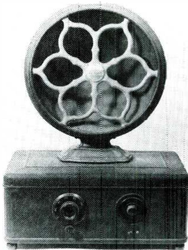
The Atwater Kent Model 52 represents the first generation of "plug-in" sets. Most sets of this era were purchased with the manufacturer's matching speaker.
