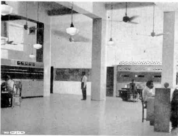
The Transmitter Hall houses two 50 kw, dual-channel, high frequency transmitters and one 10 kw medium frequency unit.
