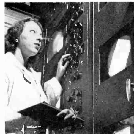
12. Final tests are made to insure that the tube will give a well-centered perfectly-focused picture.
