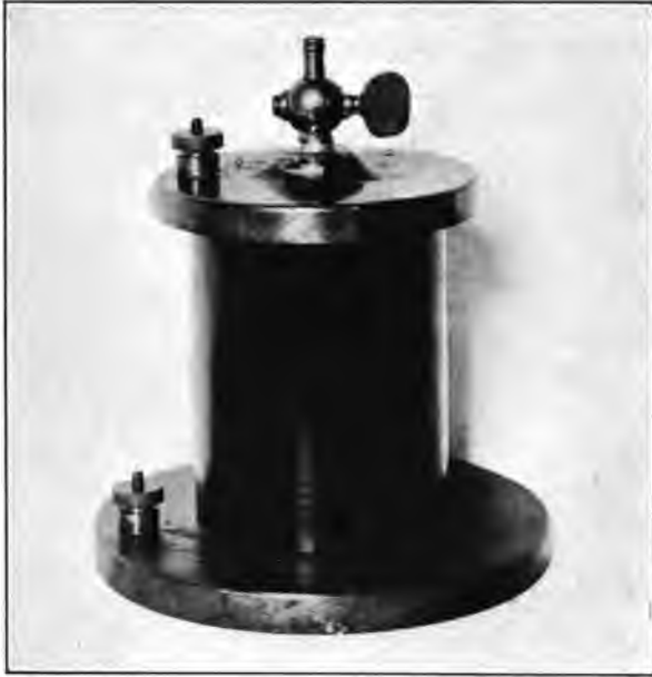
FIGURE 6—A Form of Rarefied Air Discharger for Larger Powers
