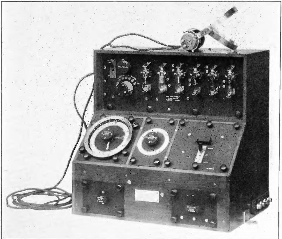
FIGURE 3—The Marconi Marine Direction Finder Type 11-B
