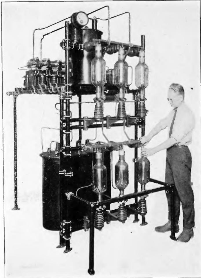
FIGURE 11—Kenotron Rectifier Unit (20-k W. Transmitting Equipment)
