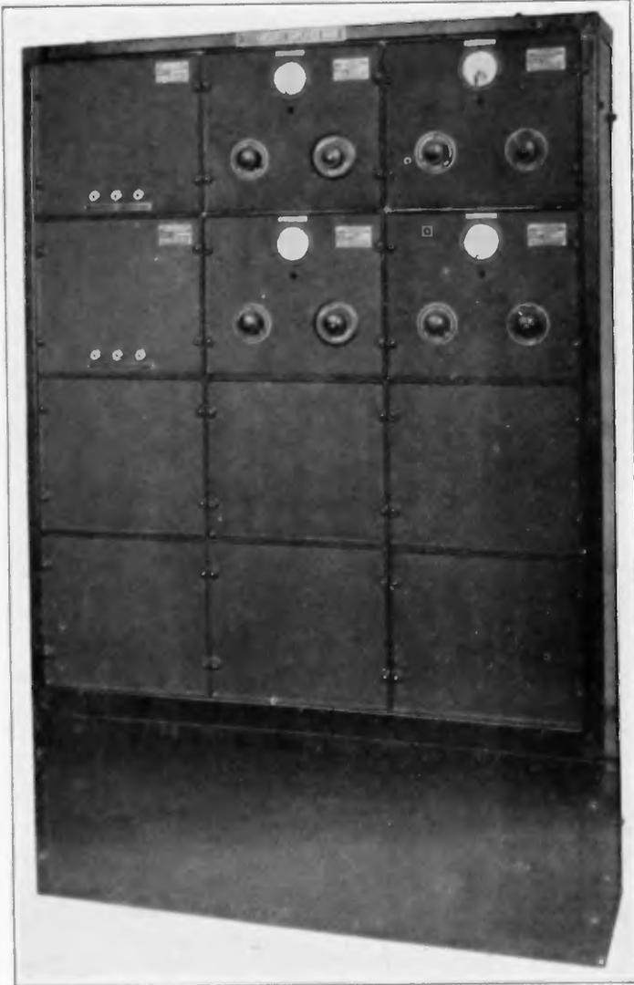
FIGURE 70—50-Watt Amplifier Rack (Intermediate Amplifier Bank) (Front)
