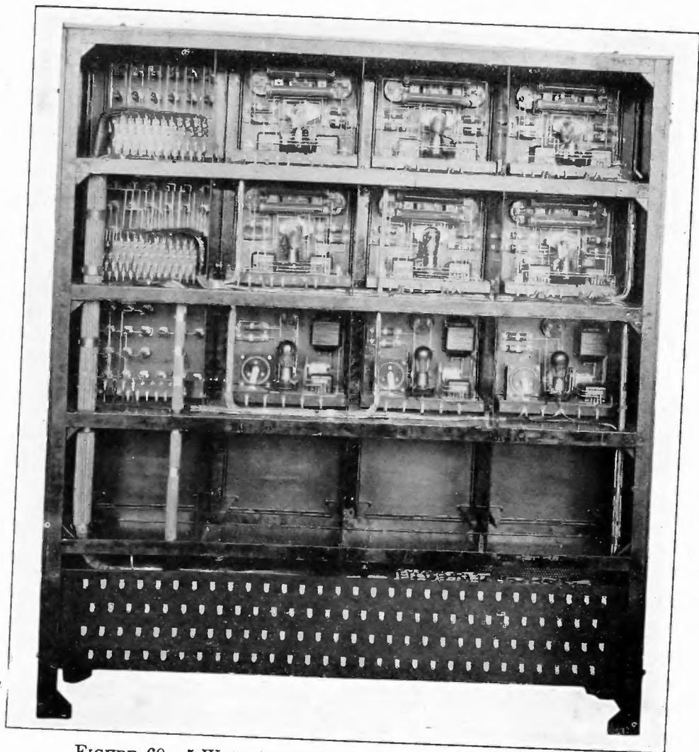
FIGURE 69—5-Watt Amplifier Bank (Microphone Amplifier)
