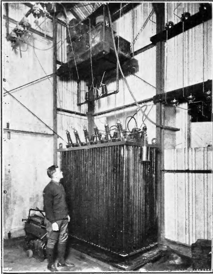
FIGURE 34—Six-phase 300-kva. 22,000-volt Transformer and Filter
