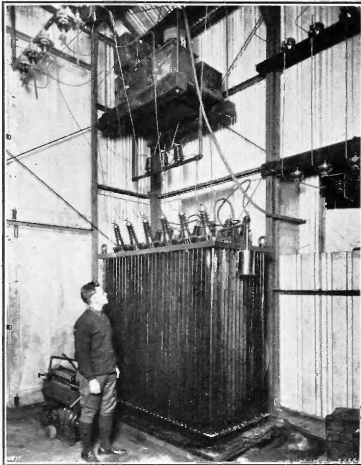
FIGURE 34—Six-phase 300-kva. 22,000-volt Transformer and Filter
