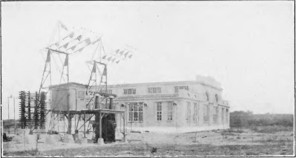
FIGURE 7—View of Radio Station and Terminal of One Antenna Wing, Station Tuning Coil, and Sleet Melting Transformers
