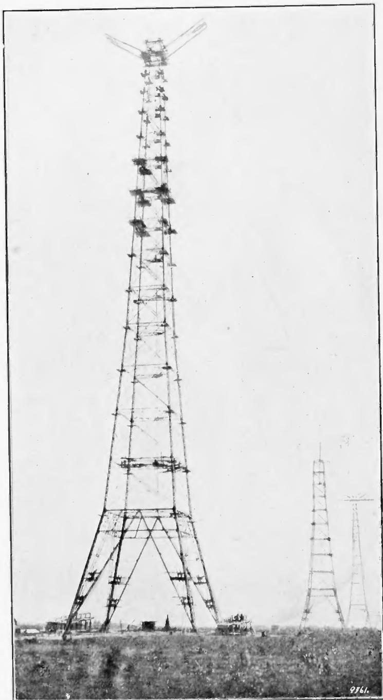
FIGURE 2—Three of the Towers in Construction Showing Cranes for Hoisting 75-foot Cross-arm Sections
