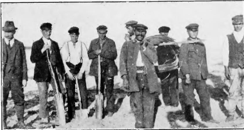
FIGURE 6—Part of Ground Laying Crew, Showing Trenching Shovels Used in Laying Ground Wire System
