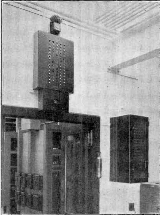
Fig. 22—Alarm Indicator and Timing Devices.
