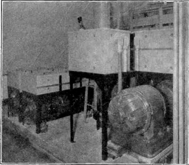
Fig. 15—Motor-Generators for D.C. Power Supply.
