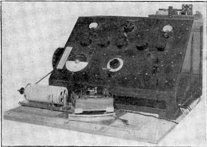
Fig. 1—Audio-Frequency Oscillator.
