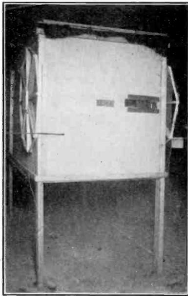
Fig. 6—Rear End of the Sound Compartment Showing the Window for Making Observations and the Octagonal Coils for Establishing the Restoring Field to the Magnet.
