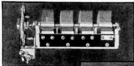
Alcoa Radio Sheet was first developed for Atwater Kent. The latest Atwater Kent condenser assembly is illustrated below.
