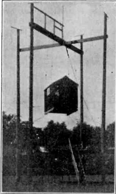
Fig. 18—View of Hut Suspended at the Center of an Adcock Aerial System. The hut contains the radiogoniometer and receiver used in taking bearings free from night errors.
