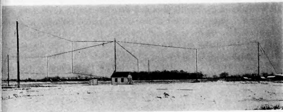
Fig. 30—Antenna system for the polydirectional radio range at Wayne County Airport, Detroit, Michigan.
