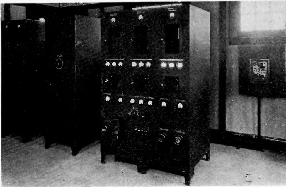
Fig. 2—General view of transmitter installation showing modulation frequency controller on the right.
