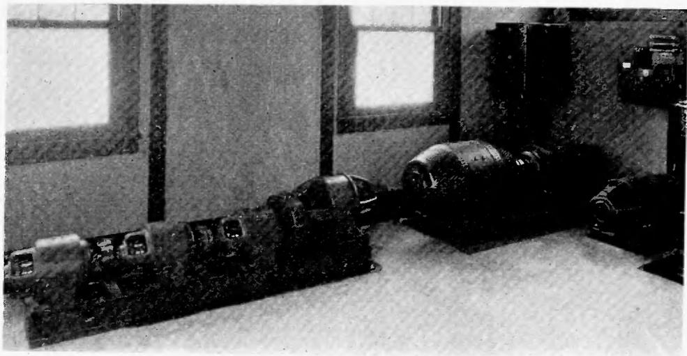
Fig. 6—View showing the high voltage generator, triple frequency machine, and low voltage d-c generator with voltage regulator.
