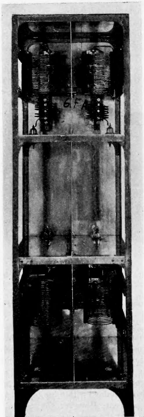
Fig. 5—Rear view of the antenna tuning unit.
