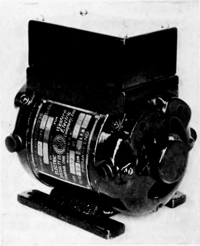
Fig. 2—Receiving dynamotor. This is driven by a 12-volt storage battery and supplies 200 volts for the plate circuit of the receiver. Weight 8 pounds.
