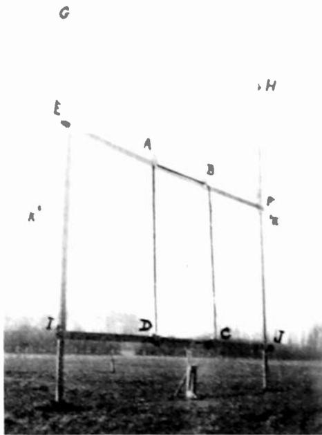
Fig. 6—View of adjustable frame aerial used for receiving.
