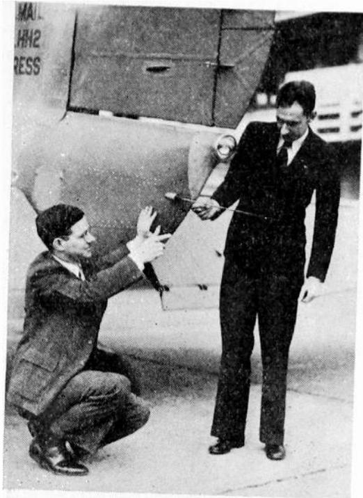
Fig. 9—Discharge point on tail of laboratory plane.
