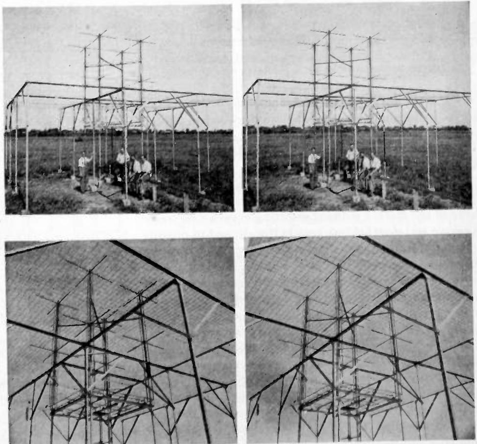
Fig. 2—Stereoscopic views of cone-of-silence marker antenna and counterpoise erected and tested at St. Hubert radio range station near Montreal.
