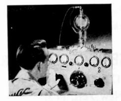
**PEAK EMISSION TESTER** measures the flow of electrons from the filaments of completed Eimac tubes. Of the long series of gruelling tests made to insure more efficient filament emission in every Eimac tube, this is the final test.
