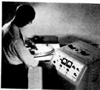
Selection of sensitivity over six different ranges can be had for measuring almost any rate of leakage. The size of the leak can also be determined with the audio system when using a helium probe at a distance from the instrument. The pitch of the leakage warning-signal changes roughly in proportion to the leak size.
