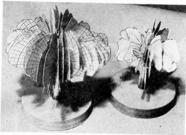
Fig. 16—Three-dimensional patterns of a one-eighth wavelength vertical antenna on top of fuselage of a B-24. Right-hand pattern is the  $E_\theta$  component and left-hand is  $E_\phi$  component.
