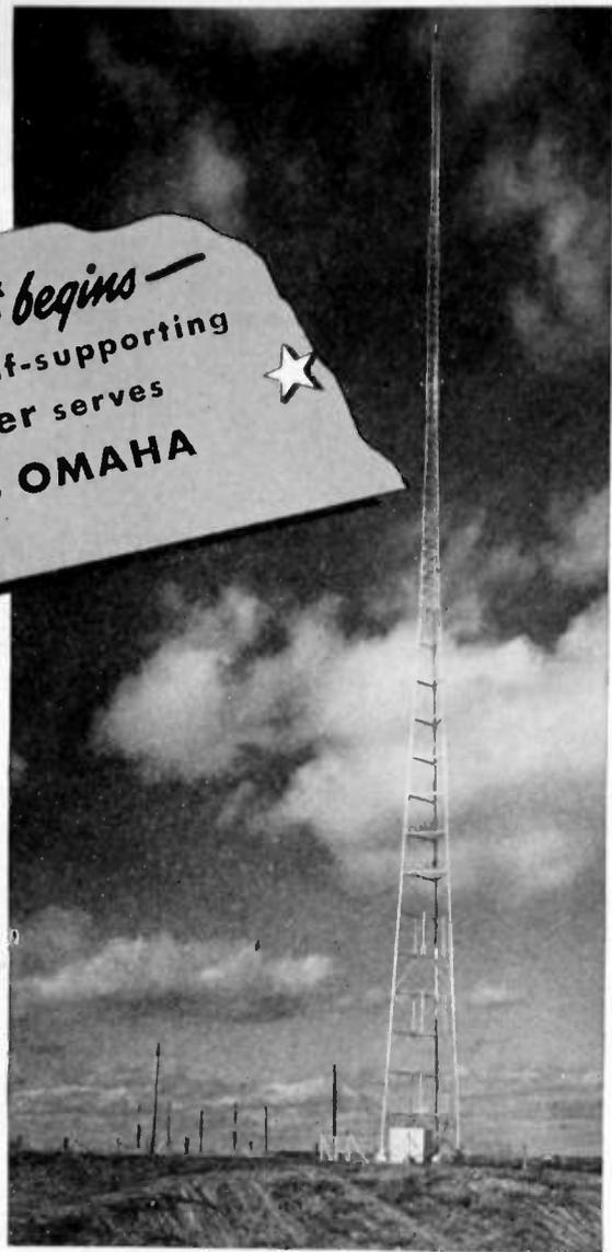
● This Truscon self-supporting tower, 300 feet high, supports an FM antenna used by the KBJY Police Radio Station at Omaha, and is one of many serving police needs in the State of Nebraska.
