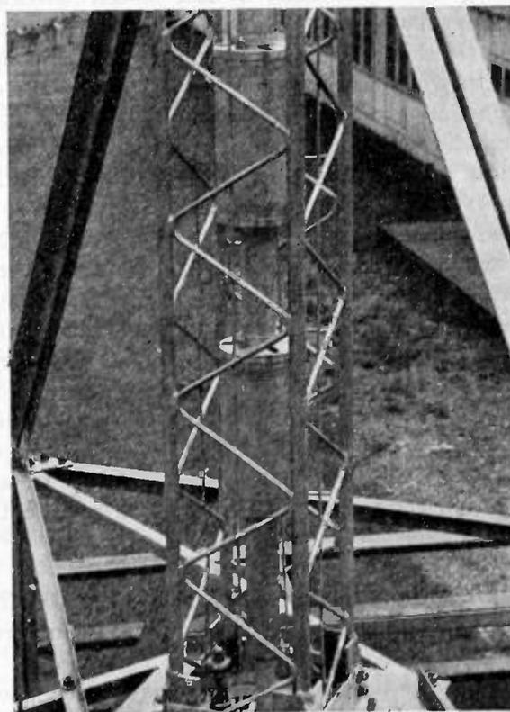
Fig. 12—Two-slug coaxial-line tuner located in the base section of a lattice-tower structure.
