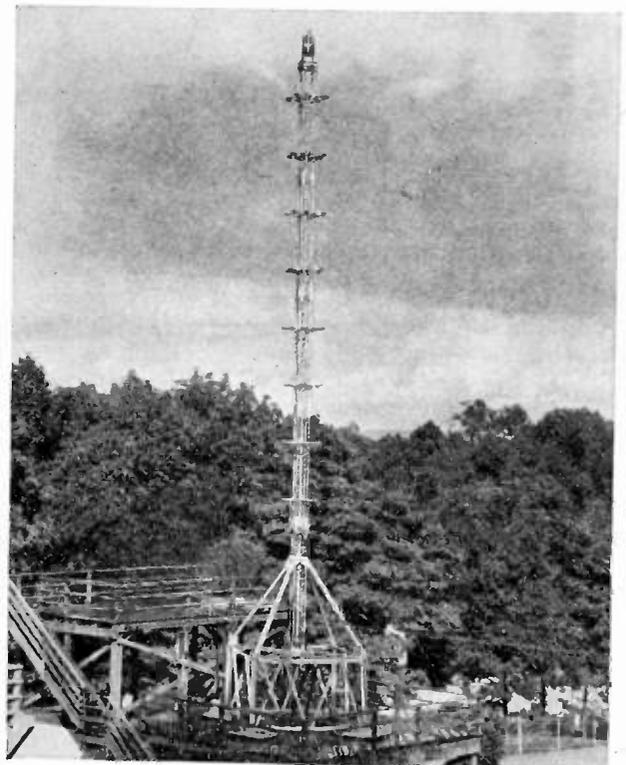
Fig. 14—A completely assembled prototype of an eight-unit cloverleaf antenna erected on a special stand for testing.
