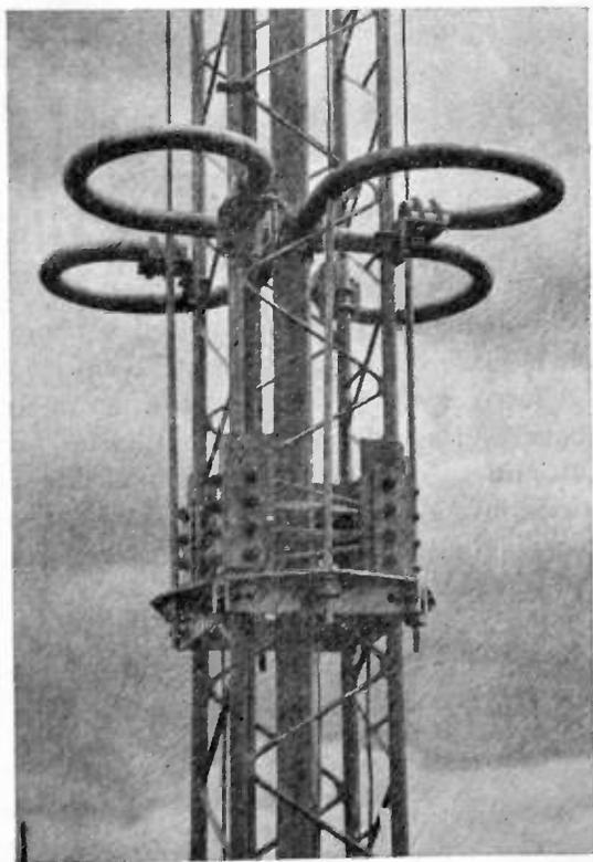
Fig. 11—Quarter-wave rods used to suppress induced longitudinal currents in the outer surface of a lattice-tower structure.
