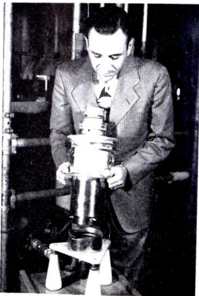
Fig. 5—Method of inserting an ML-5681 in its mounting socket.
