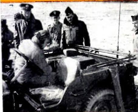
Antenna erected and power on, radio operator tunes transmitter and makes test call.
