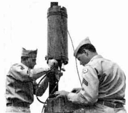
Amplifiers like this are used every 5¾ miles in the cable portions of the system. They are weatherproof, can be used on a pole or the ground, and will even work under water. The system uses a spiral wound cable developed by the Signal Corps.
