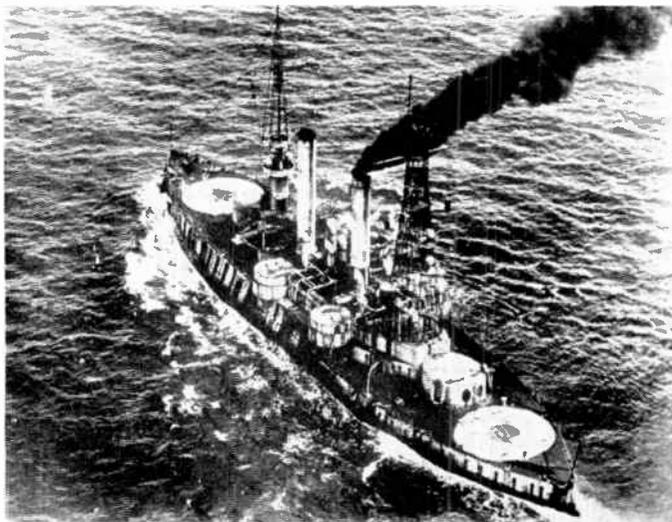
Fig. 7—The USS Iowa under radio control, 1921.
