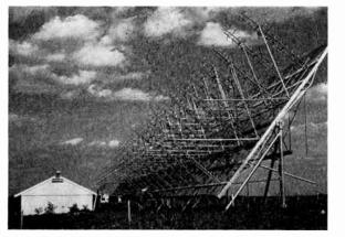
Fig. 1—Photograph of the Ohio State University 96-helix radio telescope. The antenna has a beam approximately 1.2 degrees wide in right ascension and 8 degrees in declination at a frequency of 250 mc. The telescope receiver is housed in the building adjacent to the antenna.
