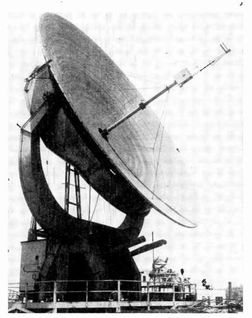
Fig. 1—The 440-mc feed horn and receiver mounted in the NRL 50-foot antenna.
