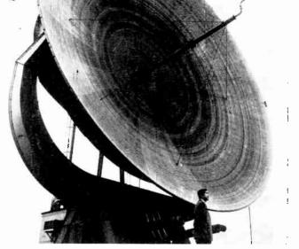
Fig. 6—Antenna used in obtaining radar echoes from the moon at S band.
