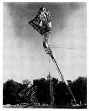
Fig. 2-Horn-type antenna feed on moon radar antenna.
