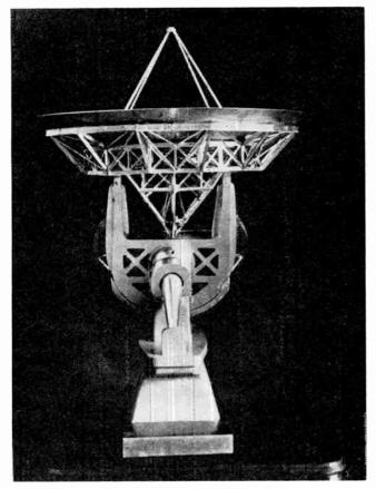
Fig. 6—Photograph of a model (about 1:60) of the 140-foot telescope, built for wind tunnel tests.
