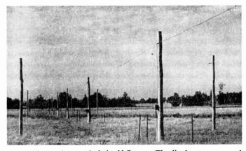
Fig.1—The northern end of the N-S array. The dipoles are supported by wires, broken up by insulators, running along the sides of the array. Nine of the boxes containing the dipole phasing switches can be seen on the poles in the middle of the array. There are 51 of these boxes in the complete array.
