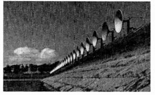
Fig. 1—The first 32-element interferometer at Potts Hill, near Sydney.
