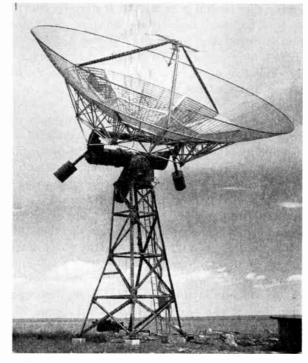
Fig. 3-One of the two 40-foot paraboloidal reflectors.
