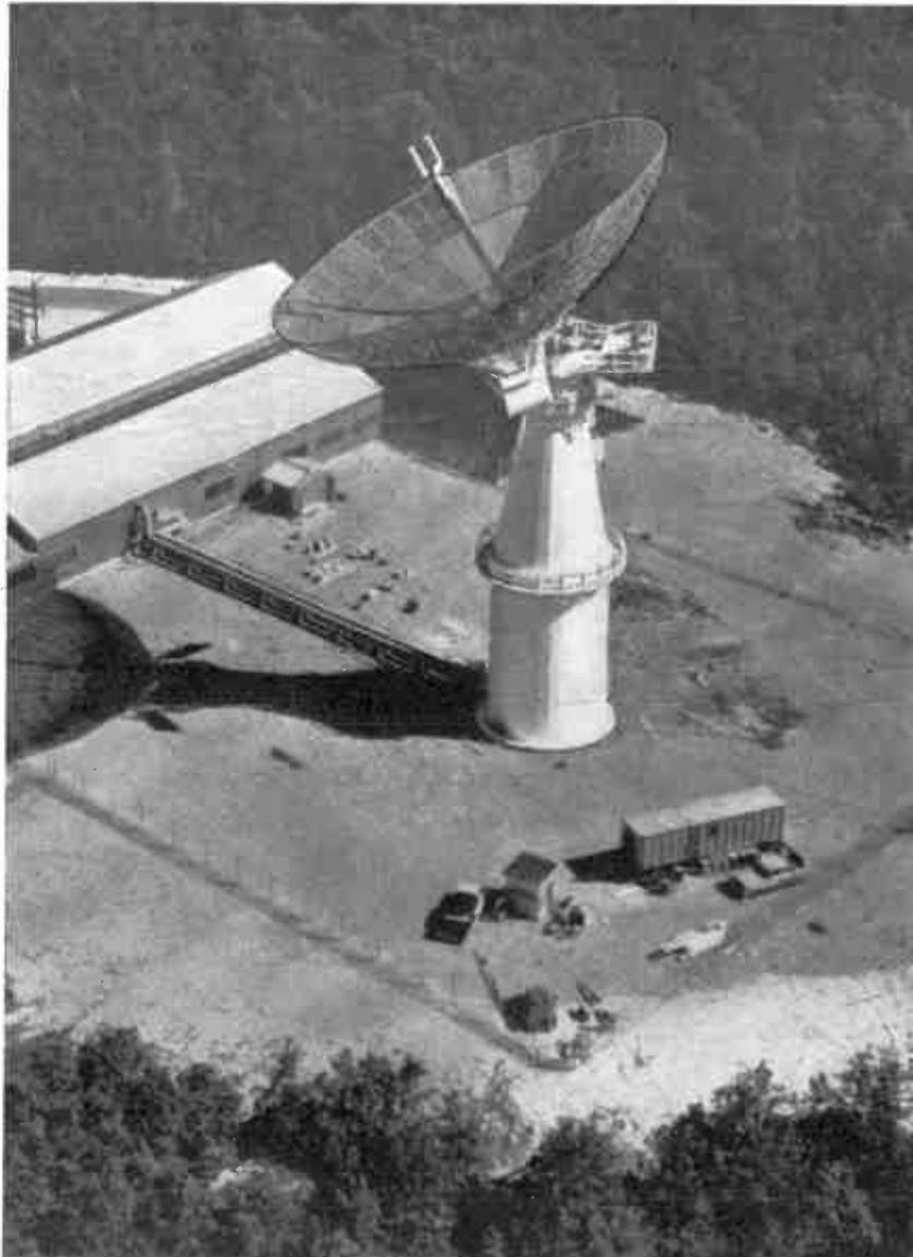
Here is the 84-foot diameter space antenna used to establish contact with the planet Venus — some 28 million miles distant. Built by D. S. Kennedy & Co., it is installed at MIT's Lincoln Laboratory at Westford, Massachusetts. Microwaves beamed from the upturned reflector made the round trip in about five minutes.
