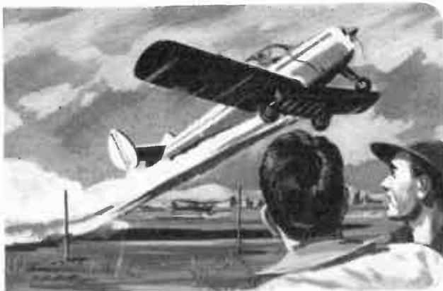
**JATO UNITS...** The nation's first successful jet-assisted takeoff (JATO) units were originated and developed in 1941 at the Jet Propulsion Laboratory, and sparked the development of future rocket vehicles.
