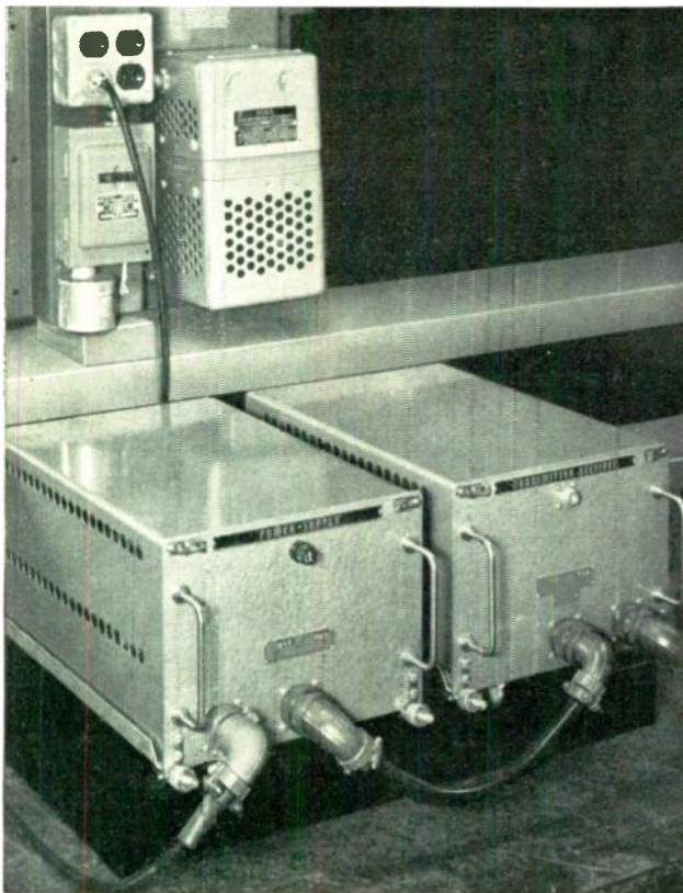
Below —Railway Communications Inc. uses Sola line voltage regulator to improve performance and reliability of this Rycom combination transmitter-receiver. Regulator delivers 118 volts stabilized within \pm 1\% under line voltage variations as great as \pm 15\% .
