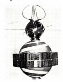
Fig. 18—Side view of LOFTI I mounted on TRANSIT III-B.
