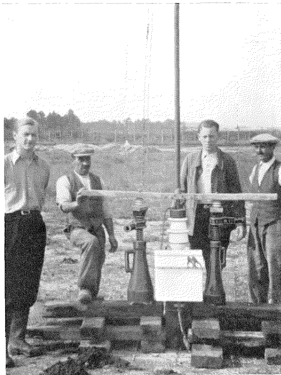
Fig. 12—Supporting Insulator and Base of Mast Aerial of Standard-Adcock Direction-Finder at Bordeaux-Mérignac.
