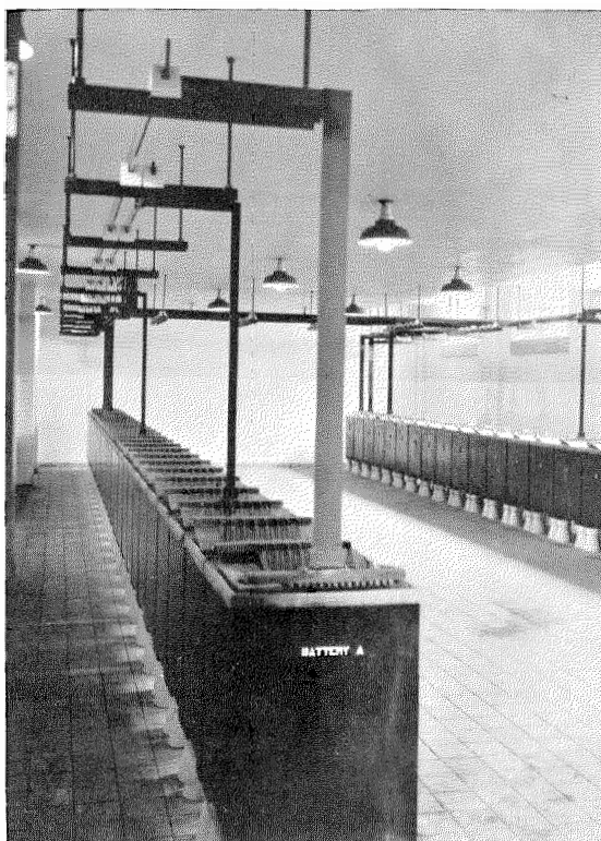
Fig. 6—Exchange "26" Battery Room.
