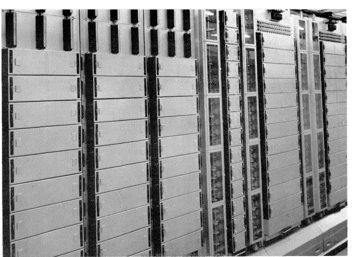
of the bay. One of these is the code sender and receiver and the other is the electronic selection control. A larger unit mounted on the lower part of the bay contains the recording and switching relays.
