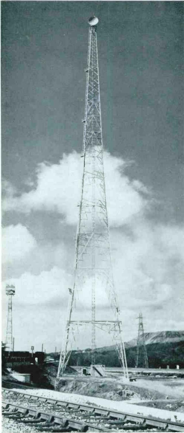
*A microwave aerial tower for British Railways' 7,000 Mc/s. multichannel link between Newcastle and York. This link, which was supplied and installed by the Marconi Company Limited, has an ultimate capacity of 300 channels and is used for telephone traffic and high-speed data transmission*
