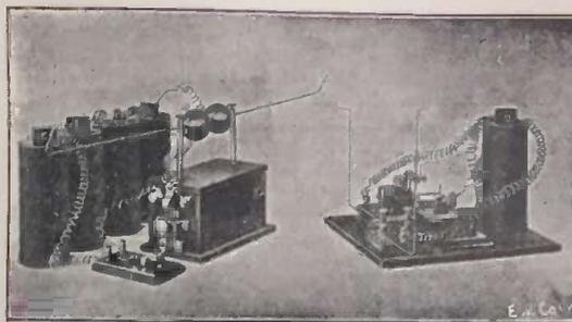
Not a toy. A scientific, high grade apparatus. Will work up to one mile. Comprises: Powerful 1-inch Spark Coil, Oscillator Balls, Key, Coherer and Decoherer, 75 Ohm. Relay, Sending and Receiving Wires, etc., etc. Guaranteed in every respect. Price remarkably low.
