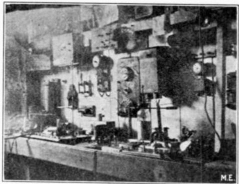
A telegraph sounder relay and lightning arrester is used, as the line runs two blocks to a friend's; also a tangent galvanometer which is very delicate.
