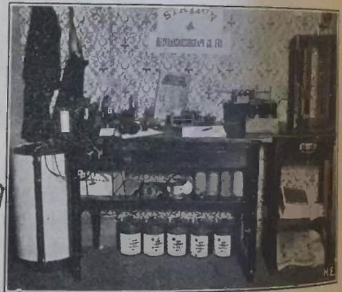
are of home manufacture, with exception of the head-phones, Morse key and induction coil, which is an E. I. Co. coil of one-inch spark length.
