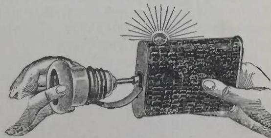
quickly prove if the lead wire inside the plug is in good condition or not.
